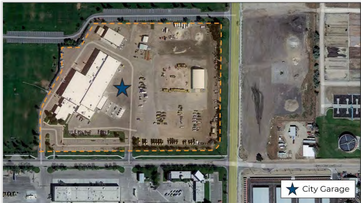
Figure 4. Aerial of City Garage Facility (1800 E K Street)
