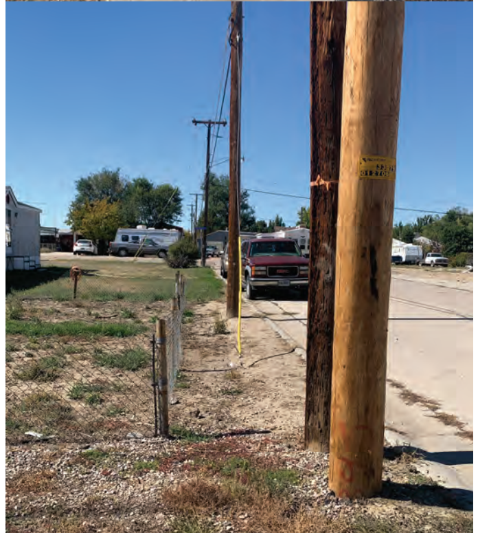
Utilities obstructing potential sidewalk
